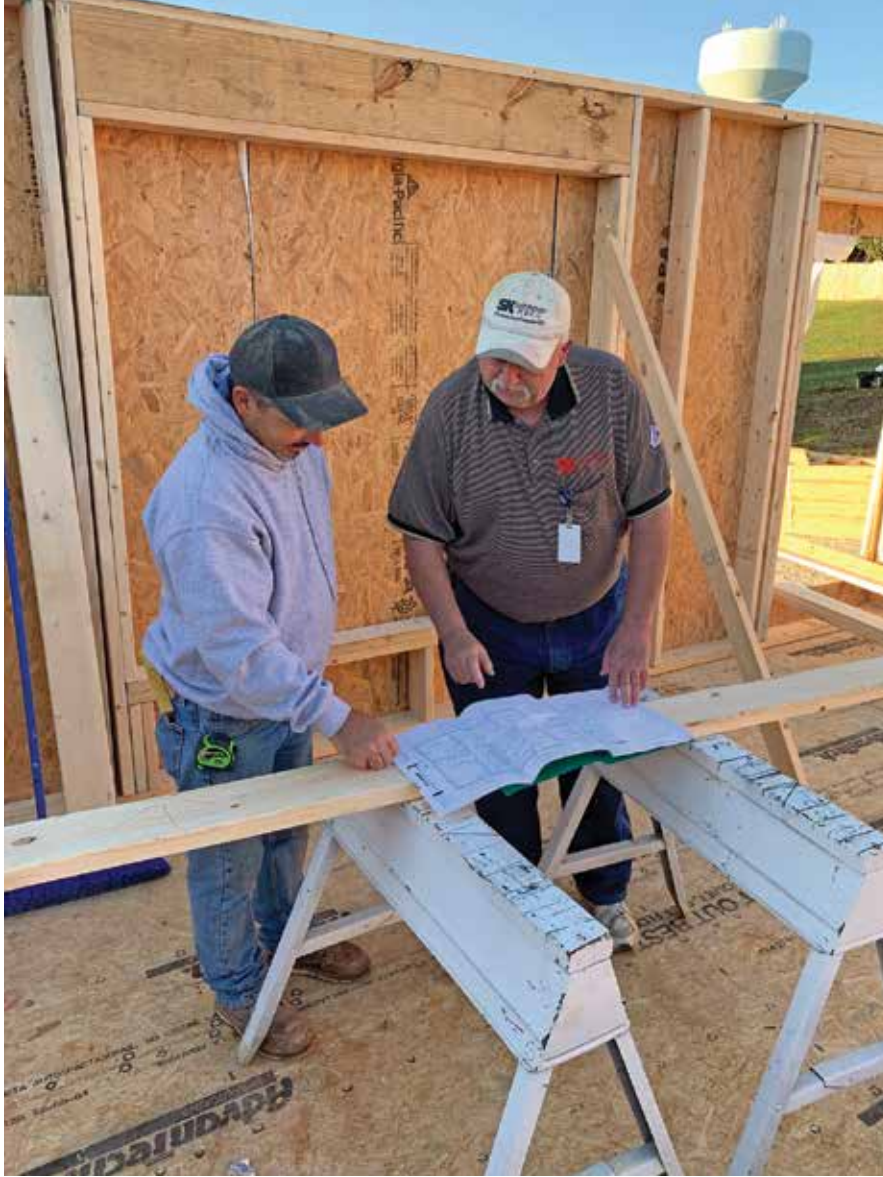
South Kentucky RECC Energy Advisor Chuck Ball works with a local builder who is constructing a Touchstone Energy Home on co-op lines. Photo: Jesse Phillips
