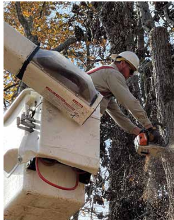
South Kentucky RECC tree trimmer Kevin Cornett is a member of the co-op's right-of-way team that works diligently to keep trees trimmed and out of co-op power lines. Photo: SKRECC Archives
