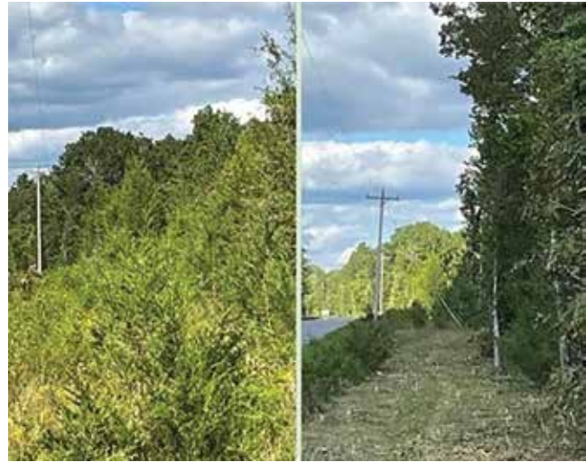
A before and after look at ROW maintenance by South Kentucky RECC's right-of-way team. The co-op maintains 7,000 miles of power lines. Photo: SKRECC Archives
